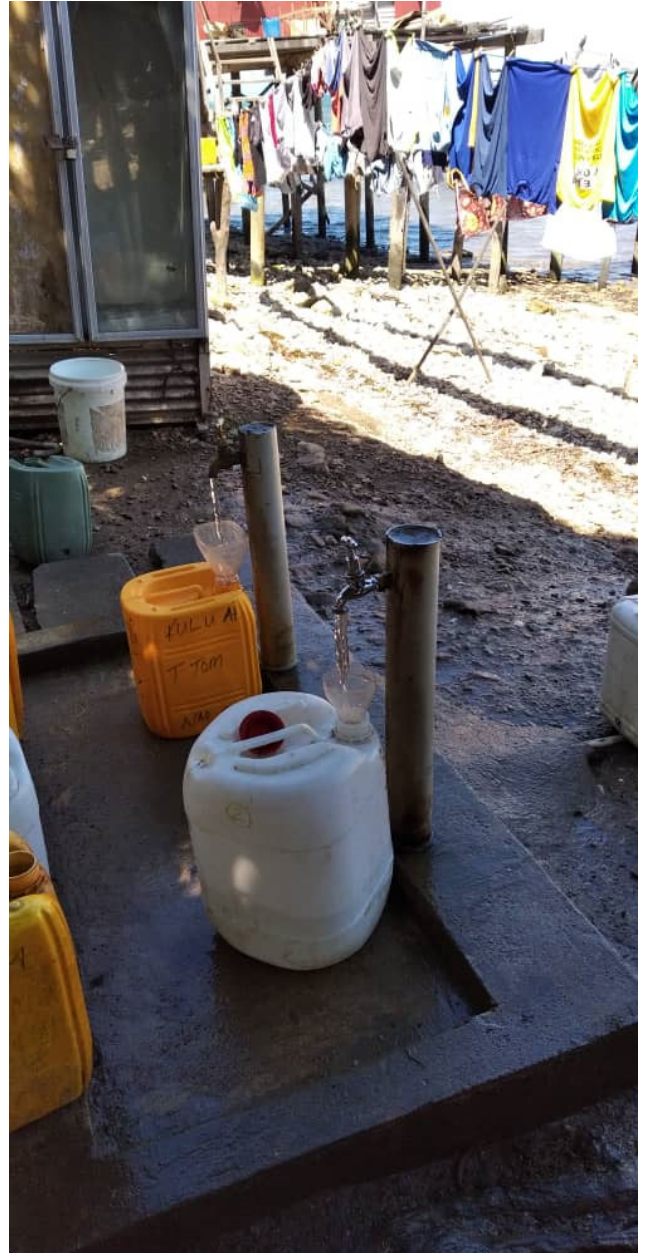
Appearances are deceptive. Water is collected from this spring and stored in large tuffa tanks and then distributed to taps.
