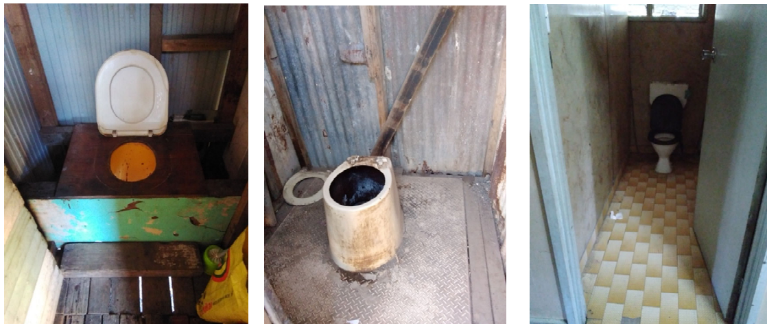
L to R: Hanging toilet, pit latrine with metal slab, flush to pit
