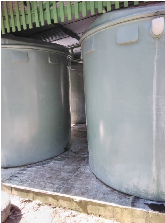
Appearances are deceptive. Water is collected from this spring and stored in large tuffa tanks and then distributed to taps.
