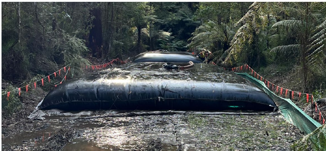
Figure 3: Sludge-filled geofabric bag.
